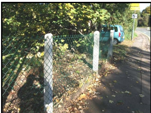
Sectional fence repair, London Road.
