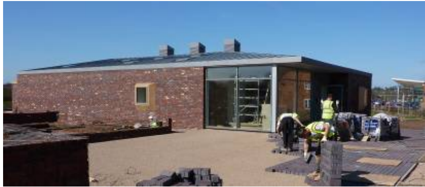
The new Darwin Park Community Hall nearing completion
