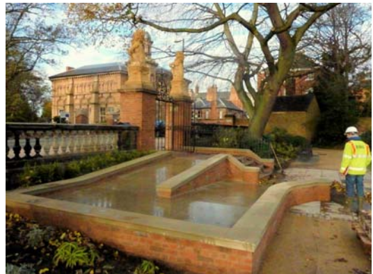
New entrance ramp at Remembrance Gardens under construction
