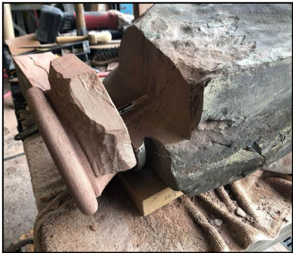
Replacement of the lower back section of stone and recarving.
