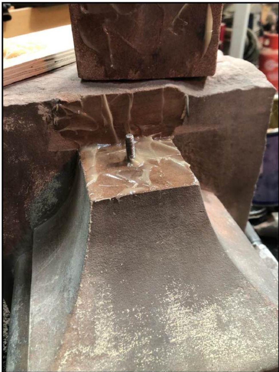
Repairs to the corbel stone.
