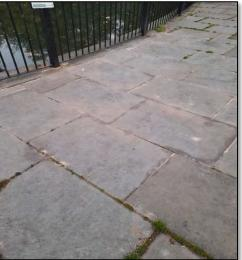
Upon routine inspection of Speaker's Corner, the granite slabs were found to be very uneven and a trip hazard. Action was taken to have the slabs lifted and re-laid as shown in the phoptographs above.
