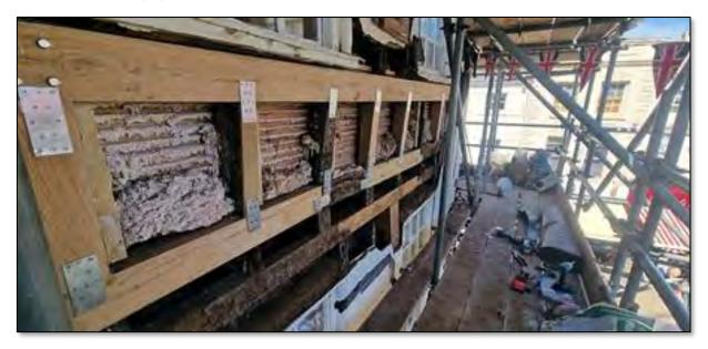
External work is ongoing at the Museum, with the new end date scheduled to be 21 October. Significant structural issues in the Breadmarket Street façade were discovered and resolved with the replacement of some beams and addition of steel brackets. At the start of September, structural work was complete and plastering underway.
