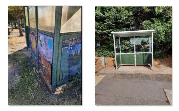
All LCC owned bus shelters within Lichfield City are in the process of being refurbished, this entails jetwashing, sanding and re-painting as a minimum, with replacement of polycarbonate and some
