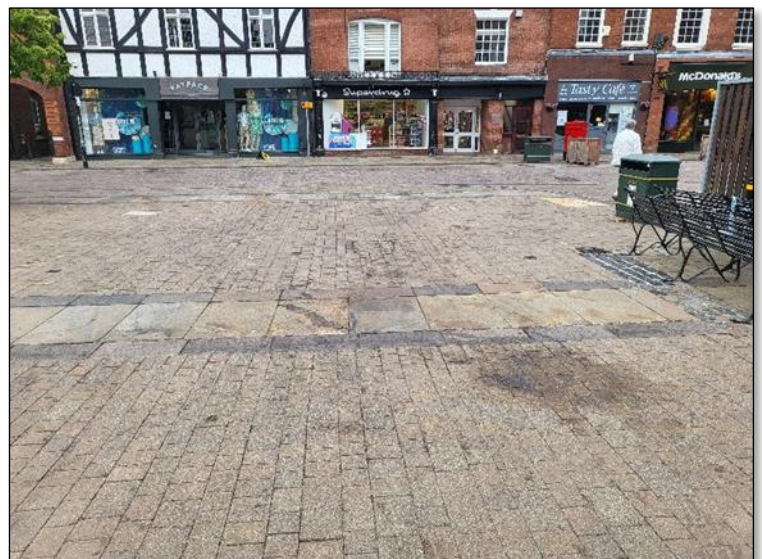
Some of the damage to the Market Square caused by oil and grease.
