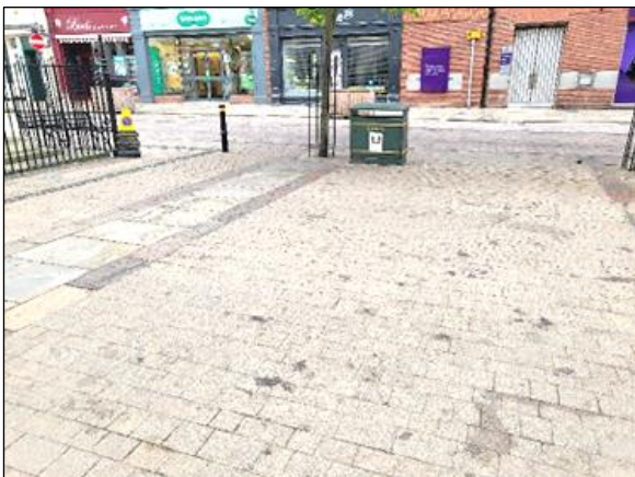
Some of the damage to the Market Square caused by oil and grease.
