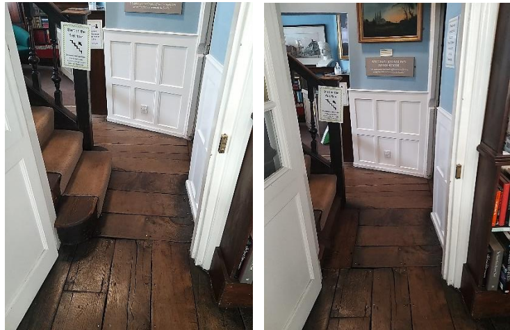
Step in usual position (shown after works completed)
